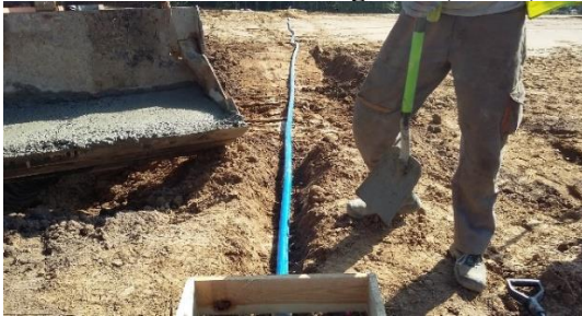
Figure 6 Profilometer profile instalation
