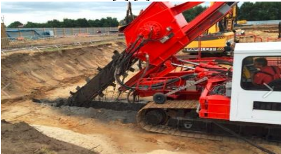
Figure 4 Trencher used in Trenchmix technology
