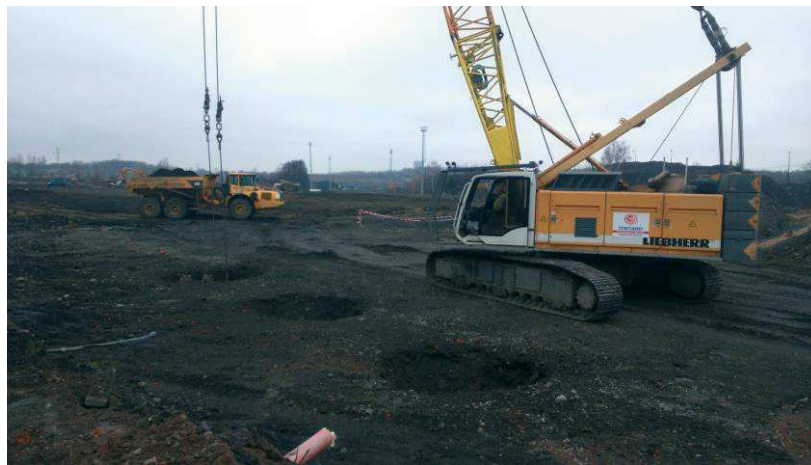
Fig. 7: Soil strengthening execution on the described project.
