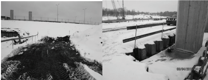
Fig. 2 Place of: a) column construction, b) measurements on the pillar
