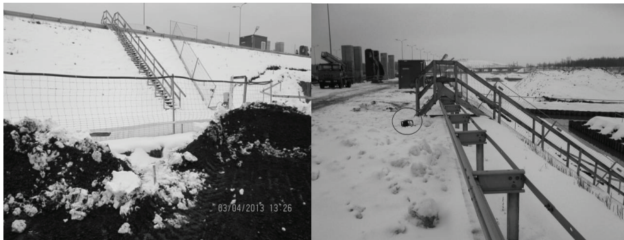
Fig. 1 Place of: a) column construction, b) measurements on the embankment
